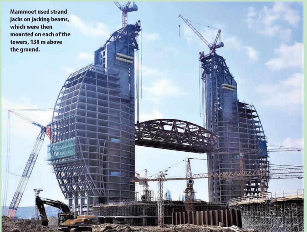
Mammoet used strand jacks on jacking beams, which were then mounted on each of the towers, 138 m above the ground.
